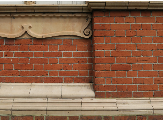
Venue 28 Brickwork Detail - Brick + Terracotta
